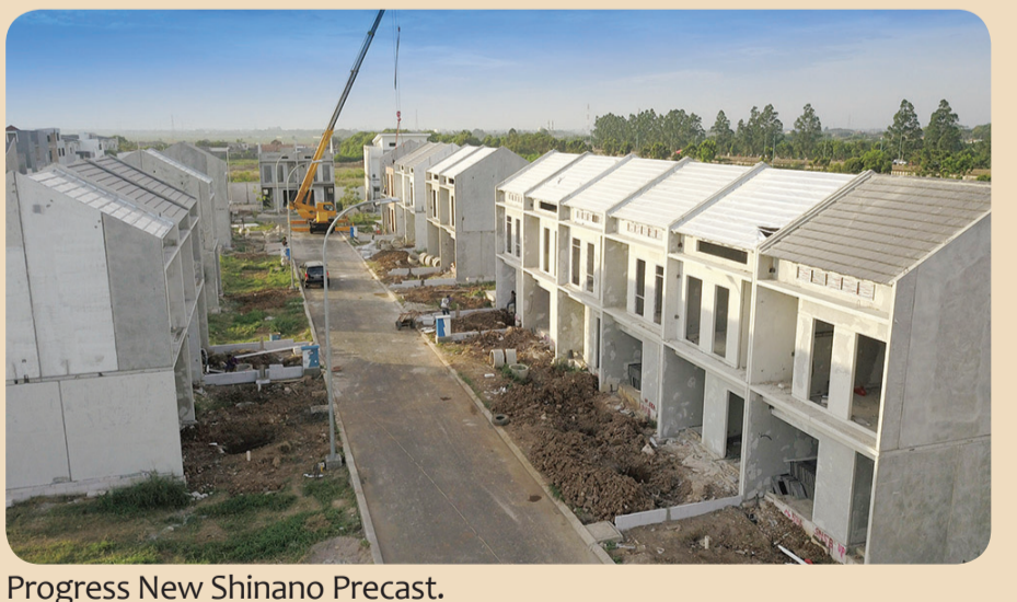
Progress New Shinano Precast.
